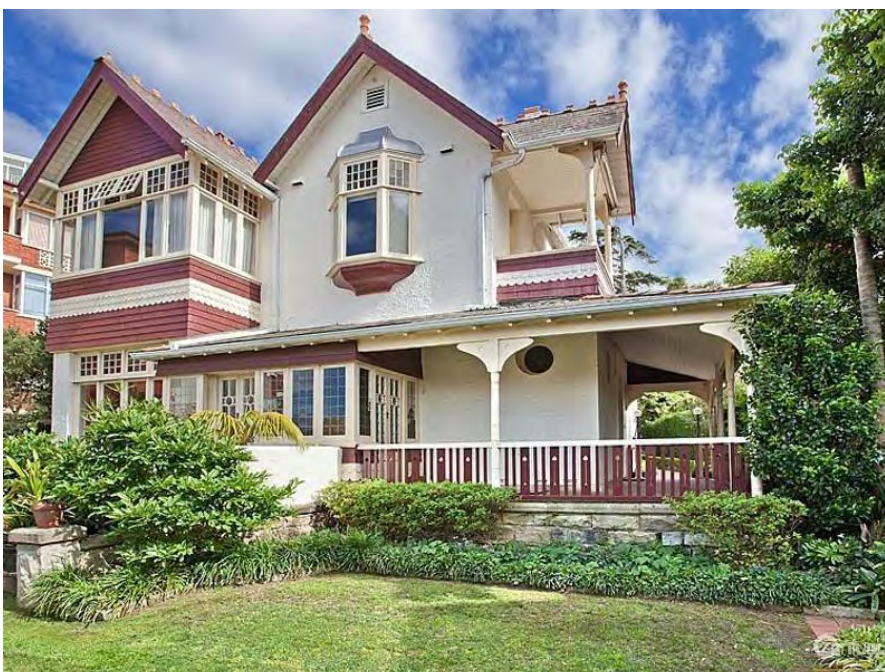
Figure 26: Photograph of Lansdowne dated 2013 ( http://www.realestate.com.au ).
