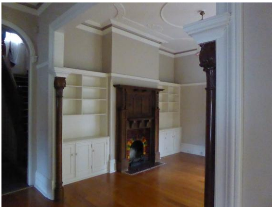
Figure 59: Chimney piece to library/music room
