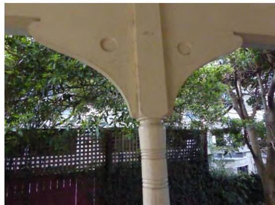
Figure 48: Detail of turned timber posts and brackets
