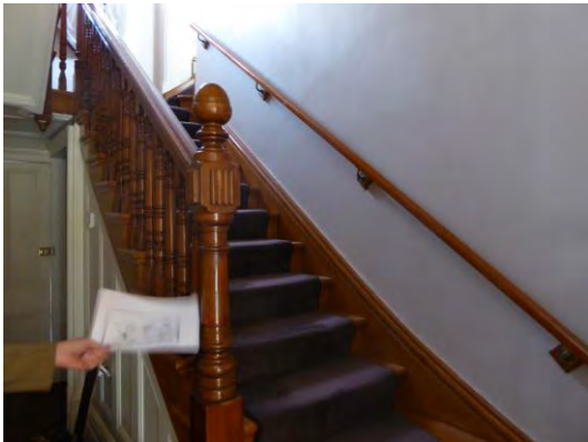
Figure 75: Original timber stair
