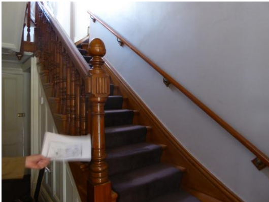
Figure 75: Original timber stair
